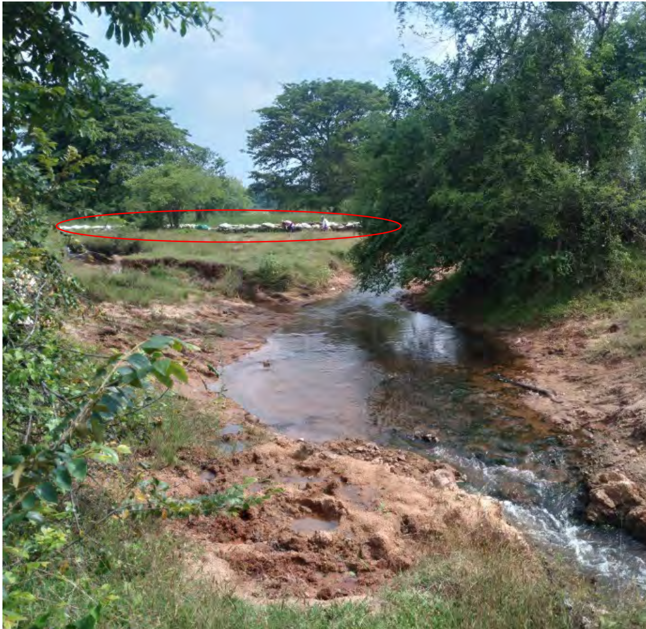
Spill canal & Spill of Kanhinddawewa. It is protected by laying sands bags (Marking by Red line)
