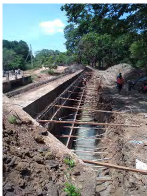
Spill construction of Meehondawewa
